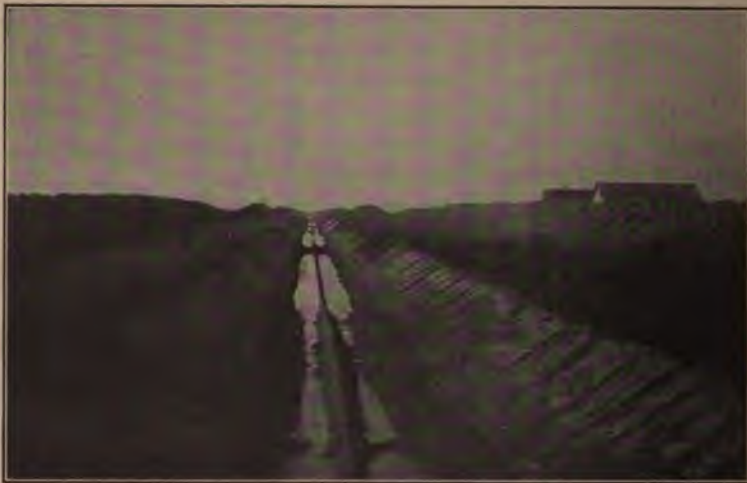
Ditch Excavated by Junkin Ditcher. Figure 62.
